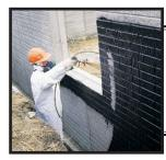
WATCHDOG WATERPROOFING is skillfully spray-applied for seamless, consistent protection against moisture.
